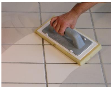
The final cleaning is done the next day with water and soap.
